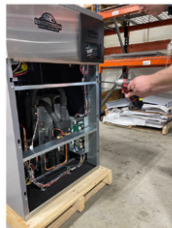
Remove three screws from the front panel to remove the side panels.
